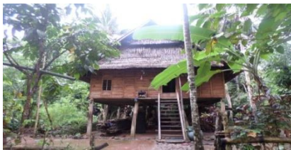
Figure 1. The house of the Kajang tribe in Figure
